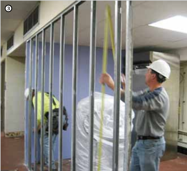
Pics from top: 1. Jim Harris at the WTC Kumm Center remodel. 2. Gary Sosalla installing metal studs at the WTC Kumm Center. 3. Jim Canar and Dennis McKee installing metal studs at WTC.
