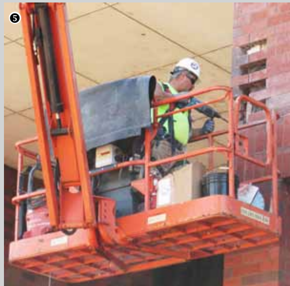
Pics from top: 1. Safety sign and eye wash station at DOIM. 3. Nick Boardman picking up rebar with the forklift at DOIM. 5. Glenn Bass preparing masonry for tuckpointing at UW-L.
