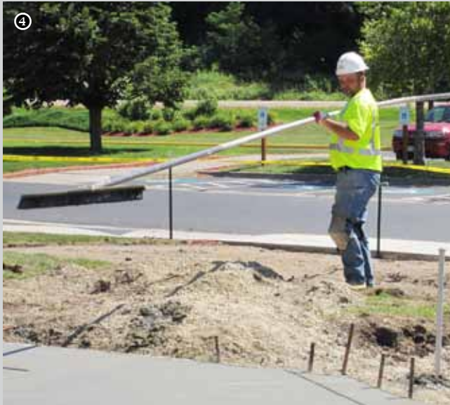
2. Andy Labelle getting the forms set up at Cabelas. 4. Troy Jacobson finishing concrete at Cabelas. 6. Sam Jaekel holding up a wall talking safety at DeSoto High School.
